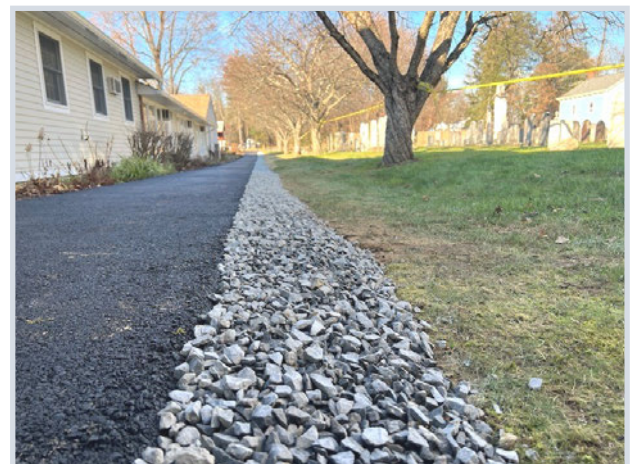
East Walkway Drainage Repair
