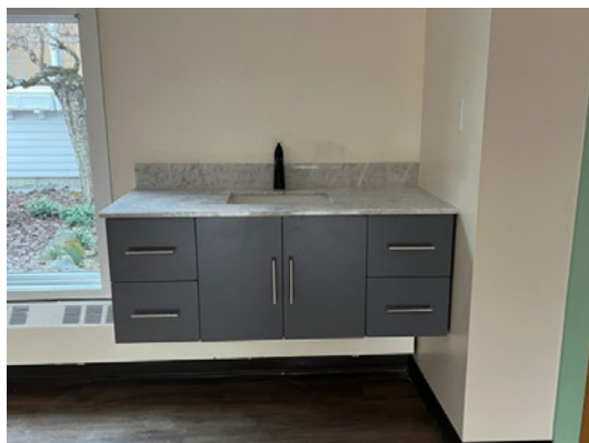
New vanity/sink in Room 7
